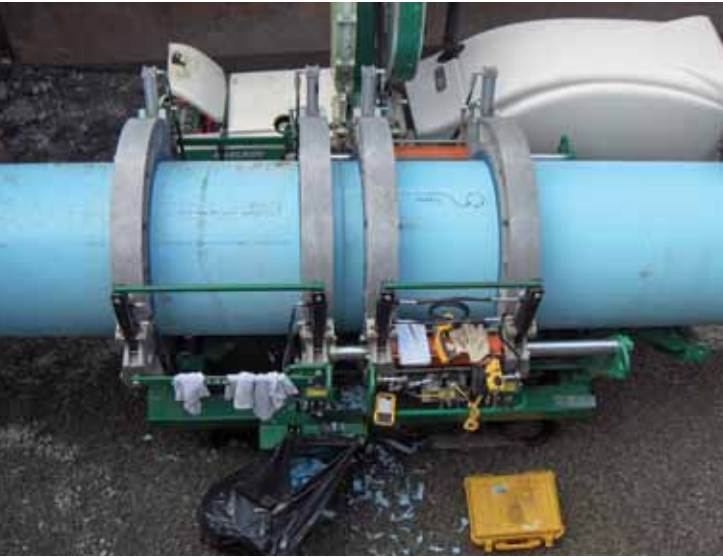
30 inch FPVC™ Pipe being fused in the pit.
