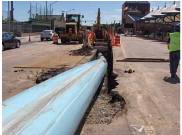
The fused section of PVC is pulled into the host pipe.
