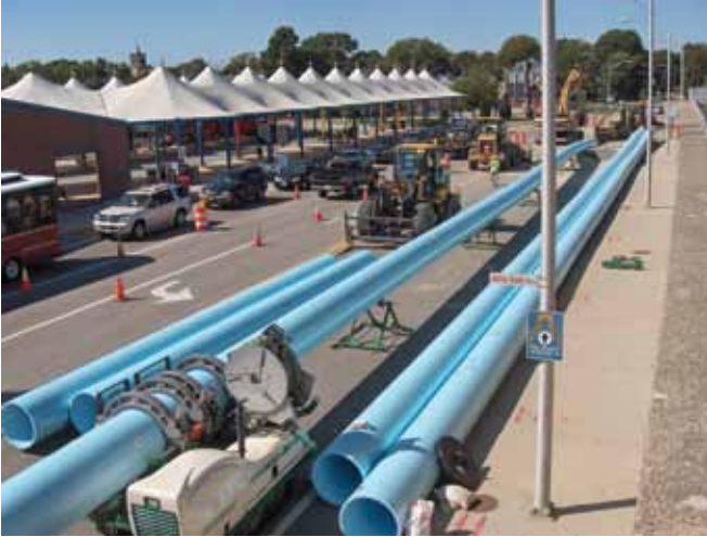
30 inch pipe ready for insertion.
