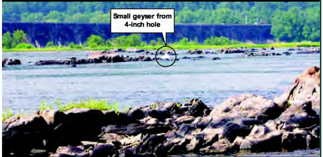
Figure 1: This small geyser appeared in the Susquehanna River in the Summer of 2005. A leak in a 16-inch cast iron line produced the geyser. It was under high pressure to help locate the leak.
