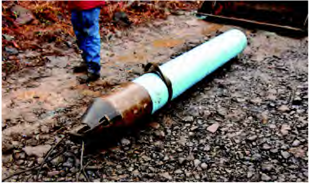
Figure 3: By pulling this "prover" through the host pipe, it demonstrated that both the pipe and pulling head could negotiate the entire run.
