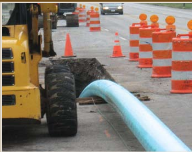
Figure 1 and 2: Example Heat Fusion Equipment for FPVCP, and FPVCP Installation in Tension via Horizontal Directional Drill
