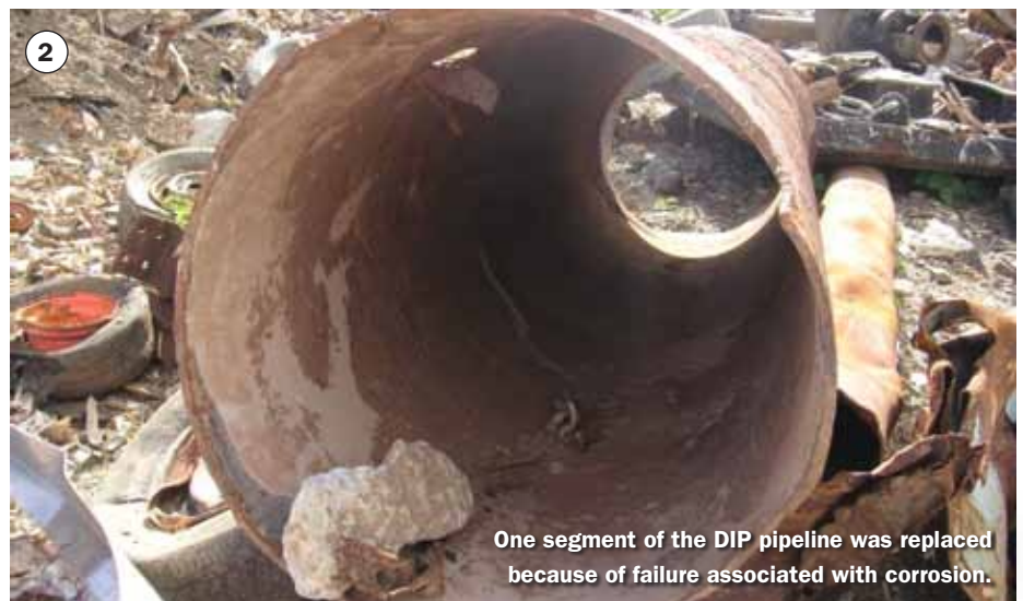
1 The original 24-in. DIP pipeline was laid in a shallow trench along the waterfront.
