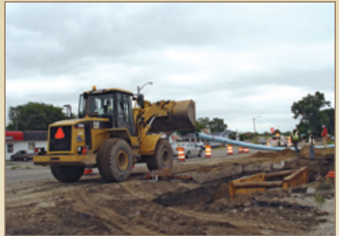
A Cat 950G moves PVC water main on the project.
