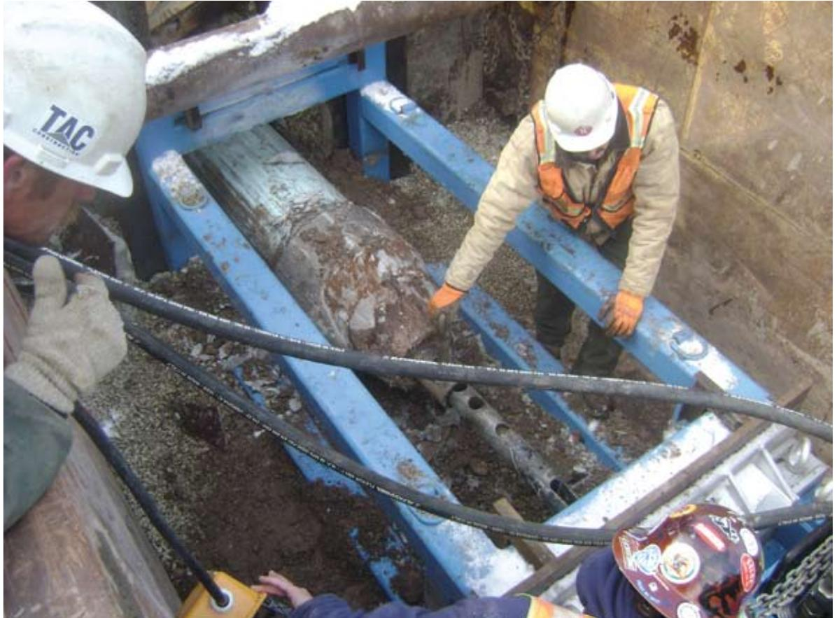
It took only four hours for the static bursting machine to burst over 800 linear feet of asbestos-cement pipe and pull in the replacement.
