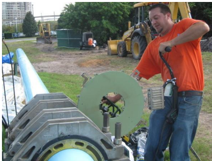
After the pipe ends have been heated, allowing proper bead formation, the heater plate is removed, and the pipe ends are brought together quickly.
